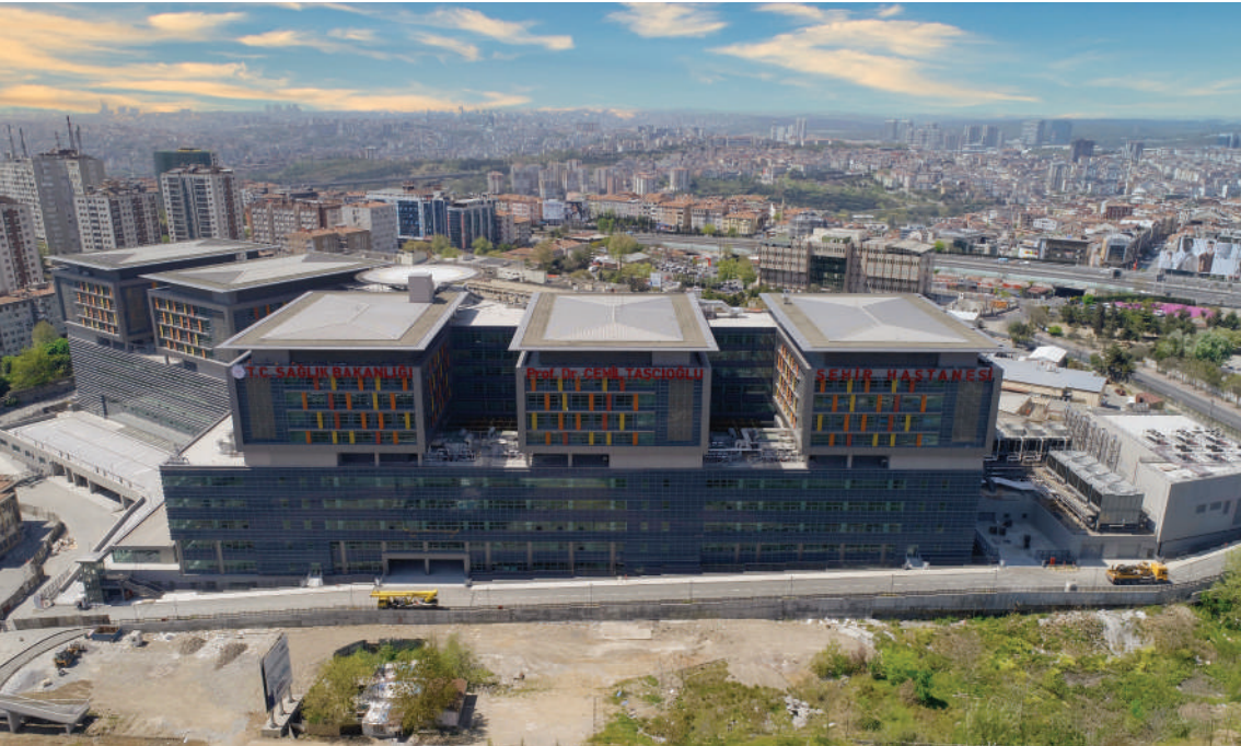
İSTANBUL OKMEYDANI (1.ETAP) ŞEHİR HASTANESİ
